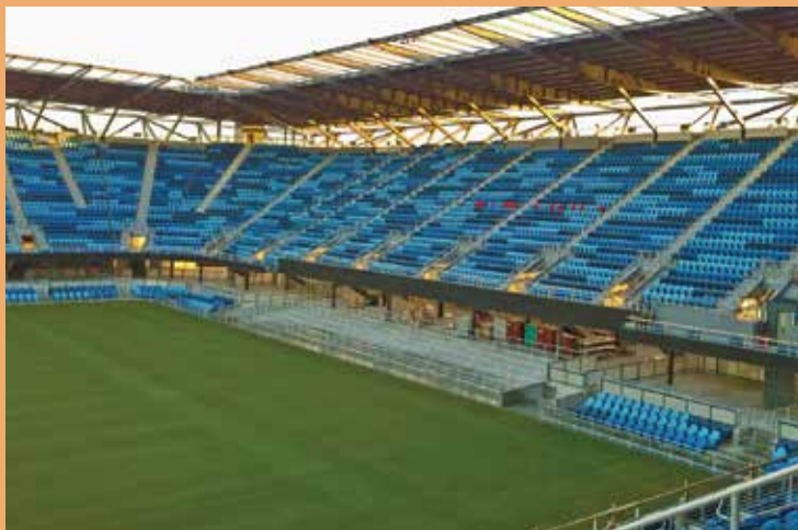
New 80-foot-long tunnel to Avaya Stadium provides safe passage for pedestrians and bicyclists.
